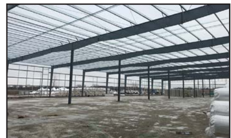
Windsor location expansion progress
