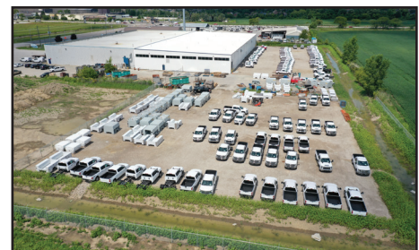
Windsor Manufacturing Facility: 85,000 sq. ft
