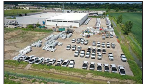
Windsor Manufacturing Facility: 85,000 sq. ft
